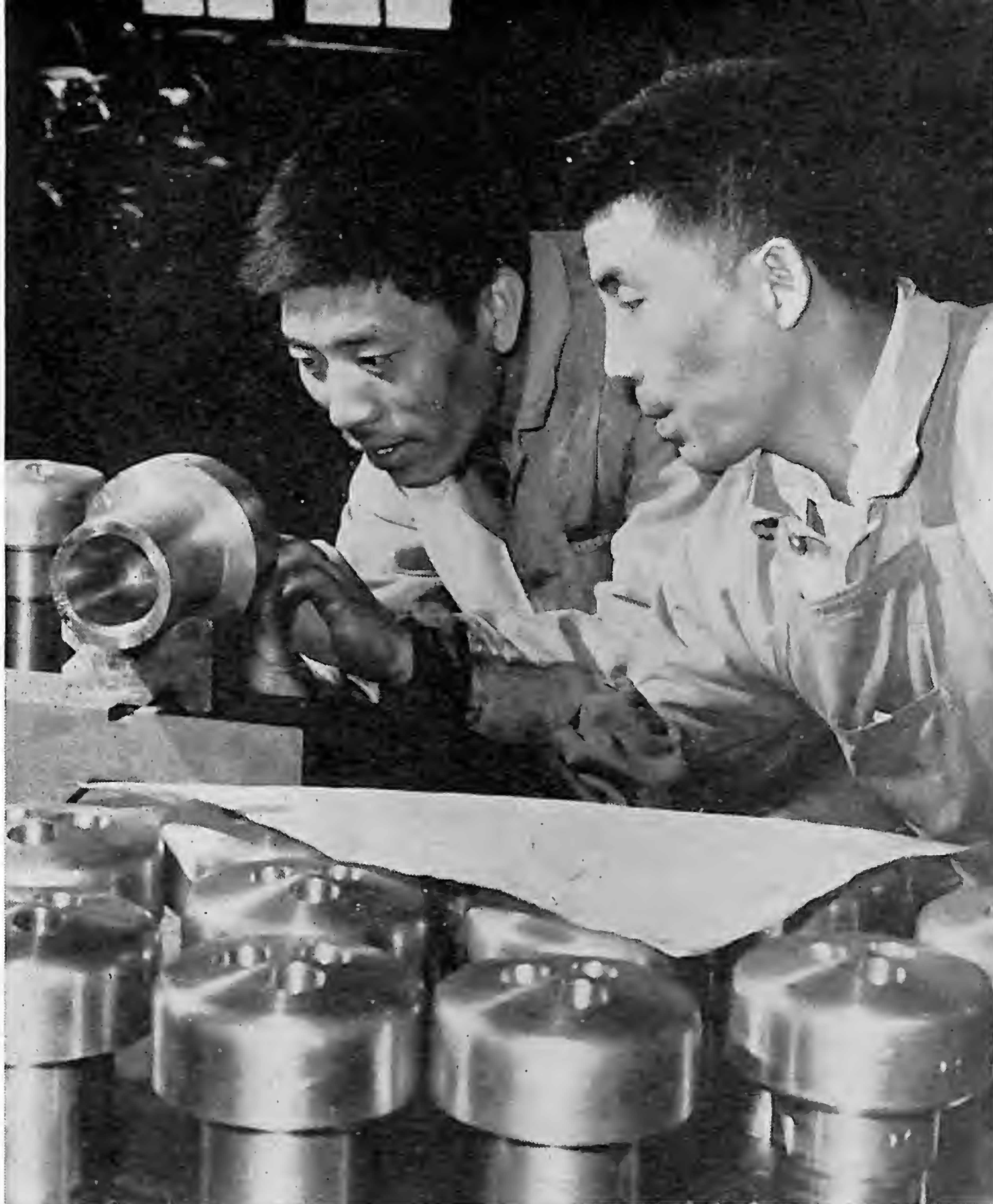
Examining the quality of the new pipe with three nozzles that blows oxygen into the converter.
